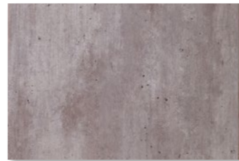
2204-K00 S Cracked Cement
