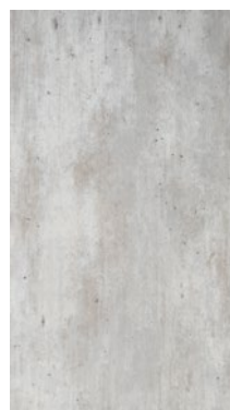
Cracked Cement 2204K00
